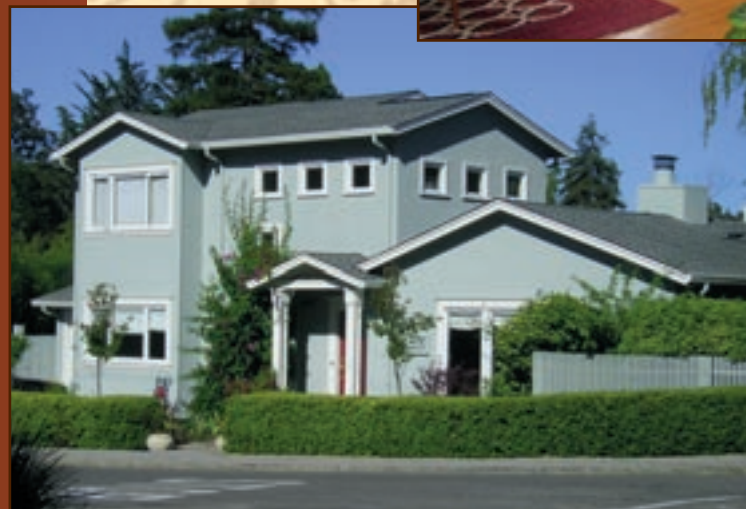
▲ Complete home remodel and addition of a second floor. —Mill Valley, CA
